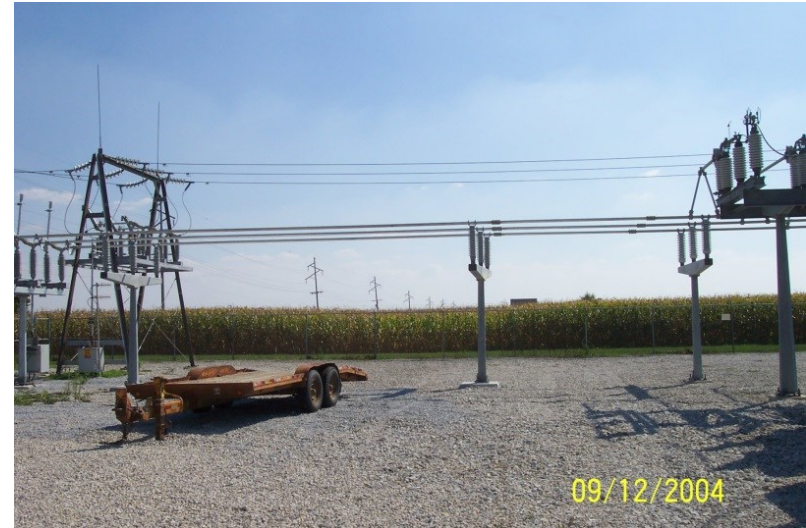
A Substation Bus
