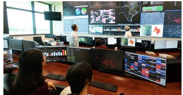
The control room at the A&M Center for Infrastructure Renewal (CIR)
