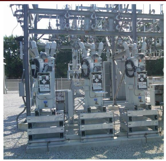
These are connected on the low side of a 69/12.4 kV transformer; each phase can be regulated separately
