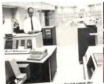
When computers were first used in system dispatch centers, they augmented the traditional analog systems. These systems were referred to as digital-directed analog control computers. As the digital computer became more reliable, it assumed full control.
