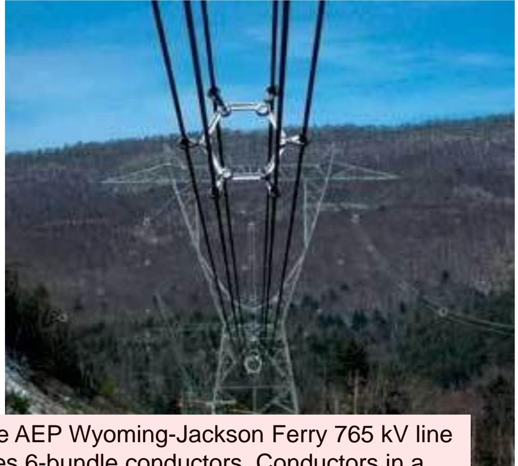
The AEP Wyoming-Jackson Ferry 765 kV line uses 6-bundle conductors. Conductors in a bundle are at the same voltage!
